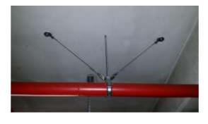
Figure 5. Installation pipes with transverse (a) and longitudinal (b) seismic isolation
